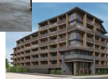
Rental condominium with hybrid structure of wood and RC BRANSIESTA MEGURO CHUO-CHO
