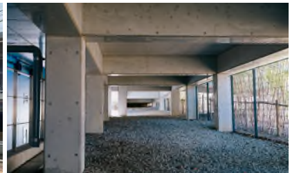
Environmentally friendly concrete "H-BA Concrete" that reduces CO2 emissions by approximately 20%
