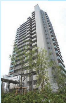
Branchera Urawa, Japan's first condominium certified as Long-Life Quality Housing
