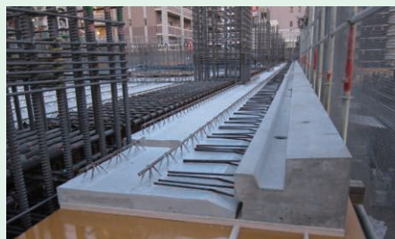
Composite precast concrete cantilever slab
