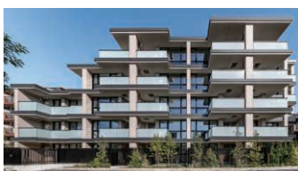
The Kensington Residence Kamiikedai
