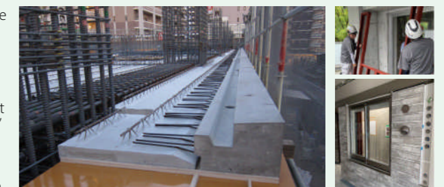
Composite precast concrete cantilever slab
