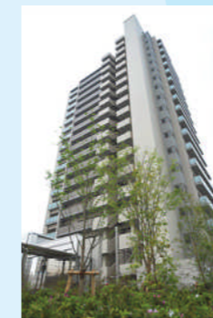
Branchera Urawa, Japan's first condominium certified as Long-Life Quality Housing
