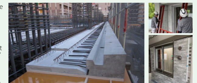
Composite precast concrete cantilever slab
